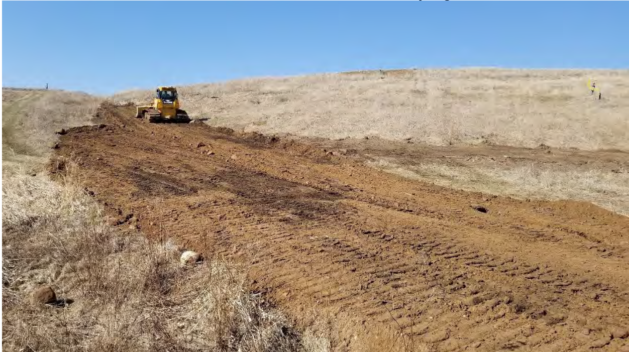
Area B south side intermediate cover haul – spring 2021
