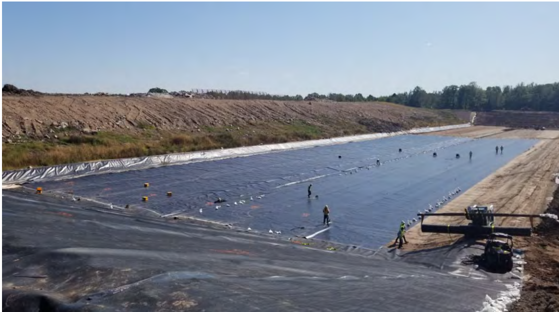
2019 Phase 5A liner installation
