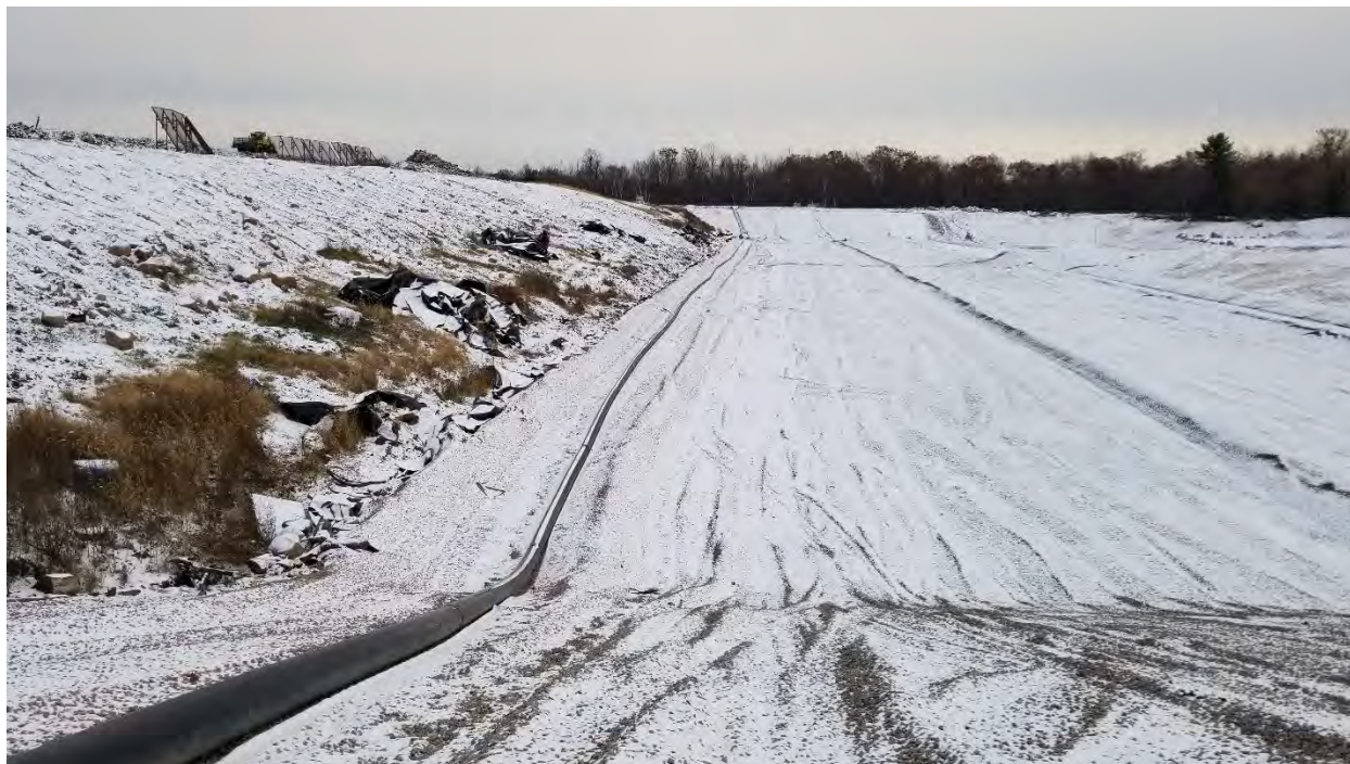
New 12" gas header along the floor of BRRDF, pre backfill.
