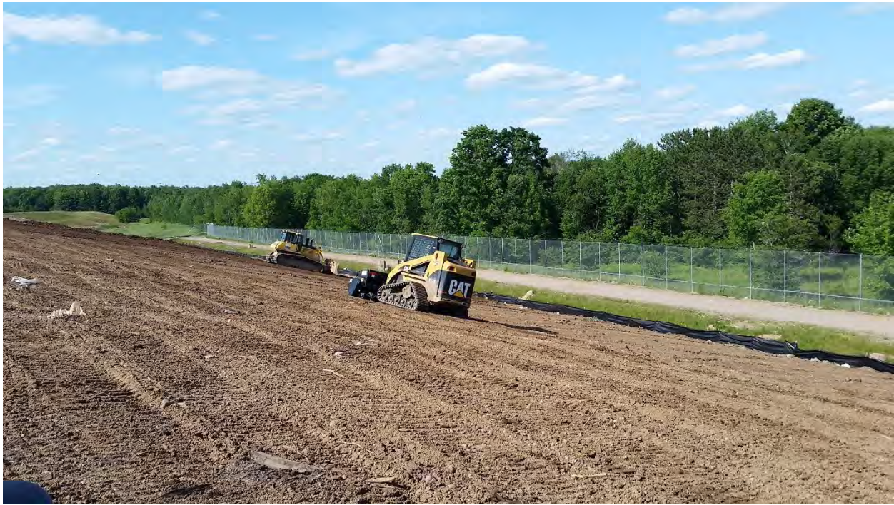
Intermediate cover grading and seeding
