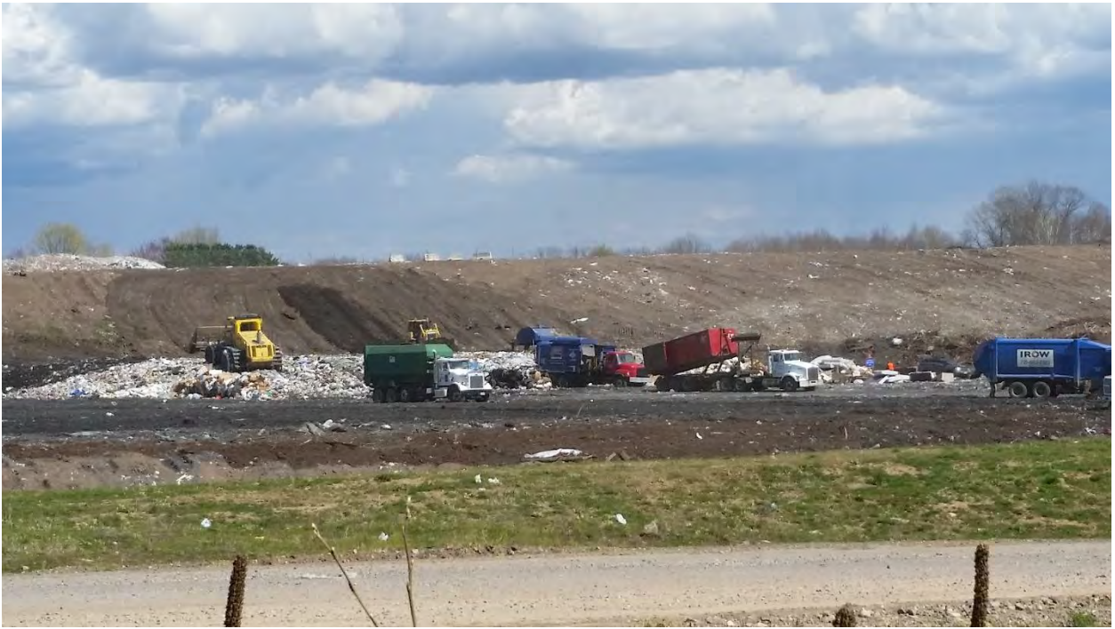
Operations, ash used as daily cover, clean soil as intermediate cover
