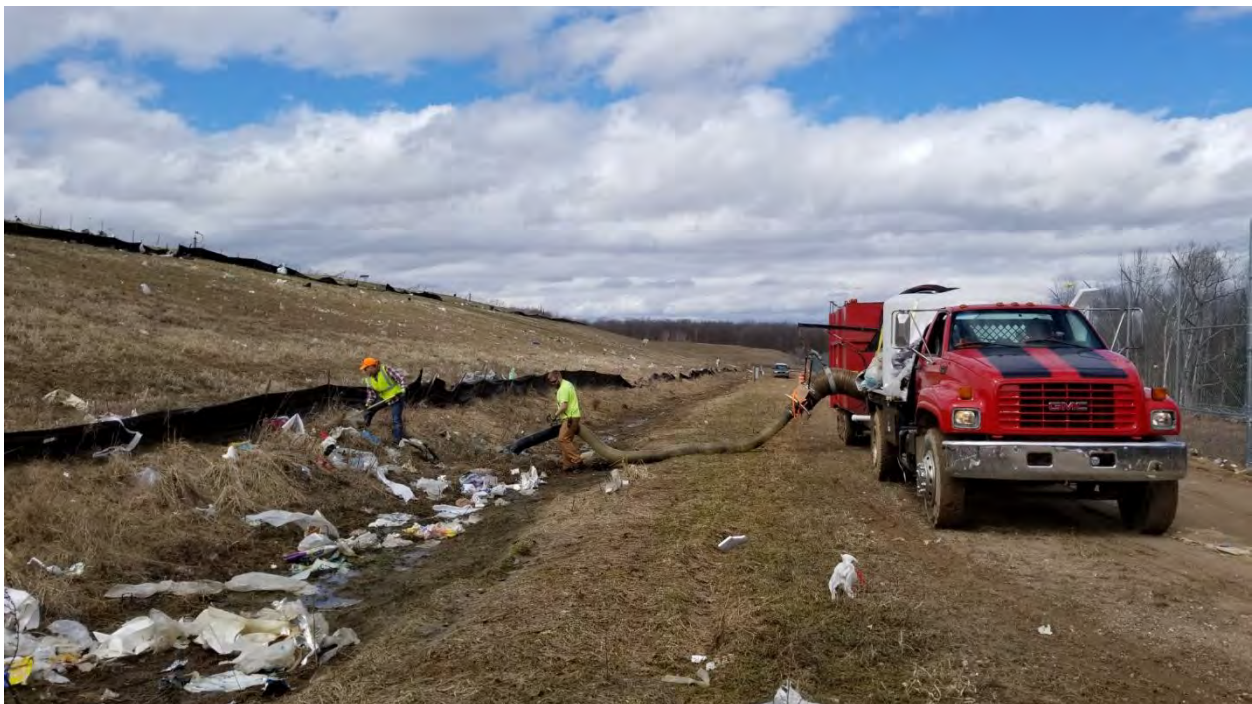
MCSWD staff working to clean ditches after snowmelt; utilization of a large vacuum
